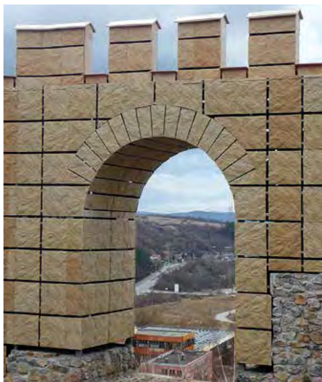
Ongoing reconstruction at Krakra fortress, Pernik
