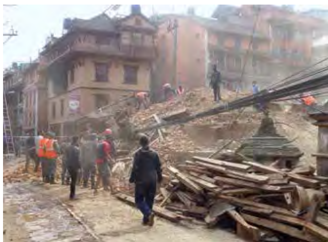
Community and armed forces helping to salvage from a collapsed temple in Patan
