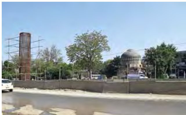
Construction of viaduct piers in front of Buddha Ka Awa
