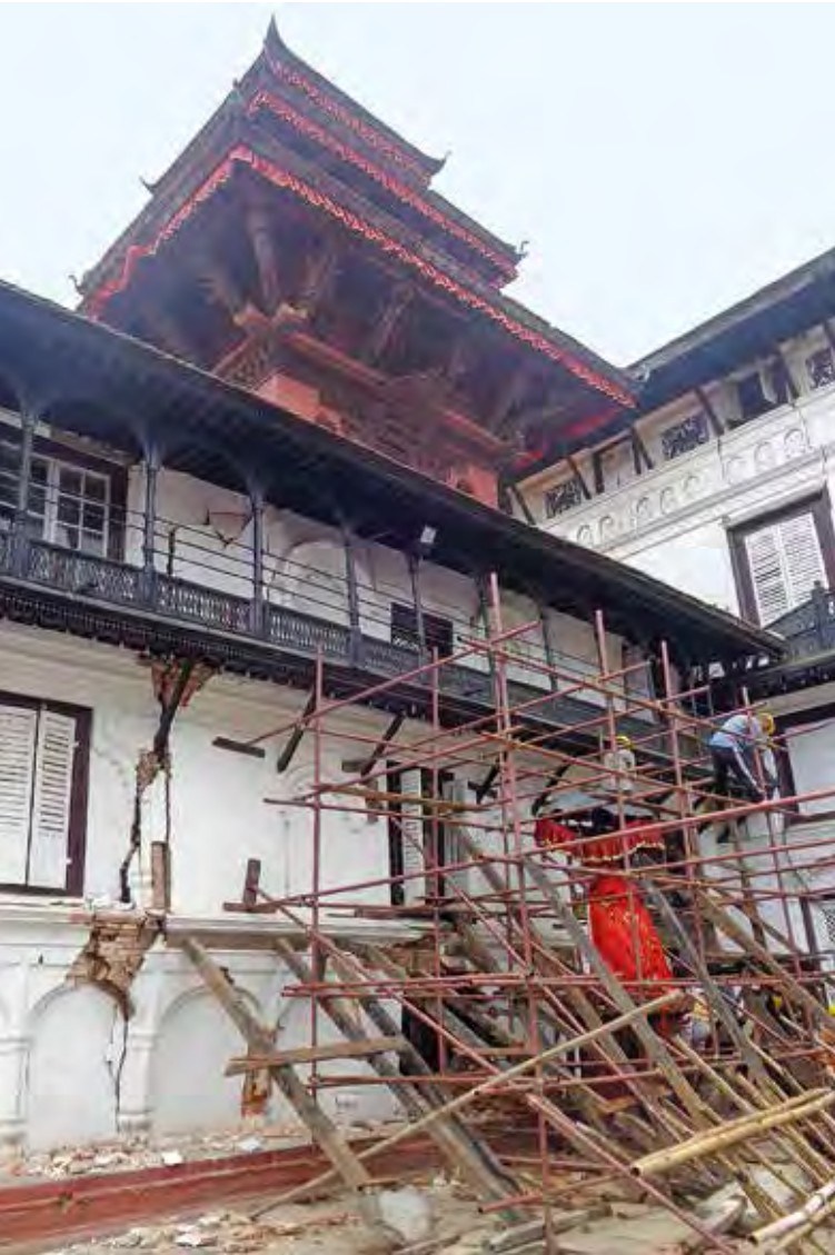
Shoring to protect the façade from collapsing onto the main Hanuman Statue with the intact Agamchhen Temple that is raised on timber stilts over the palace
