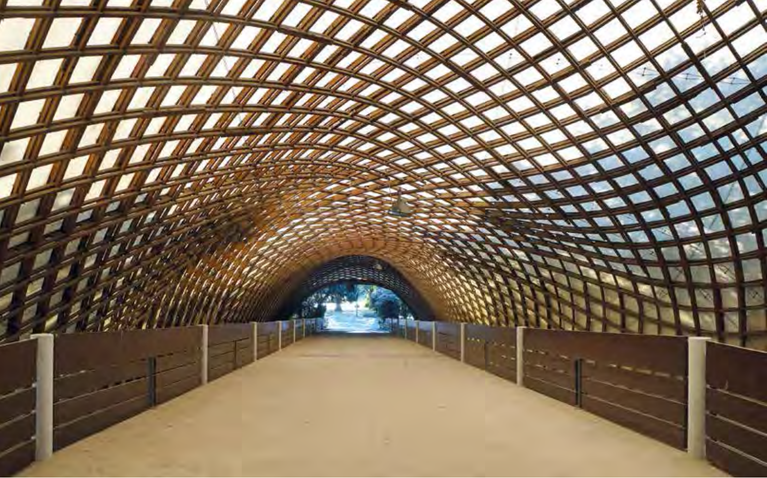
Inside view of the Multihalle (photo Architektenkammer Stuttgart)
