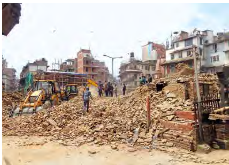
Collapsed Kastamandap, the oldest monument which gave Kathmandu its name (meaning wooden structure), regrettably being cleared using excavators
