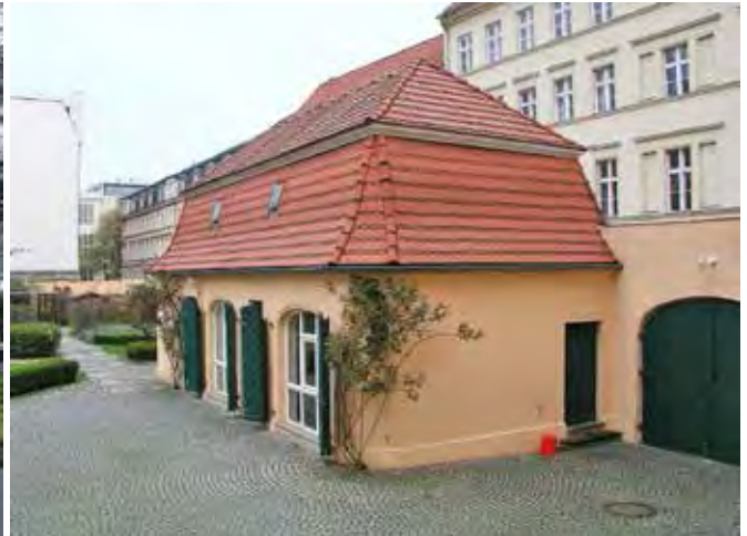
The Remise (depot-building) gives an idea of the scale of the garden
