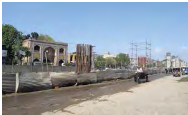
Construction of viaduct piers in front of Gulabi Bagh
