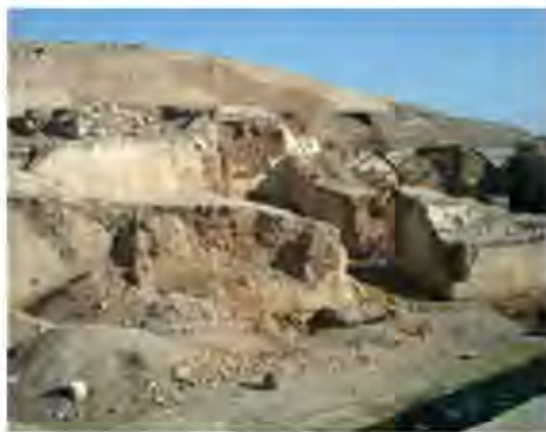
Ebla- Damages in the Royal palace
