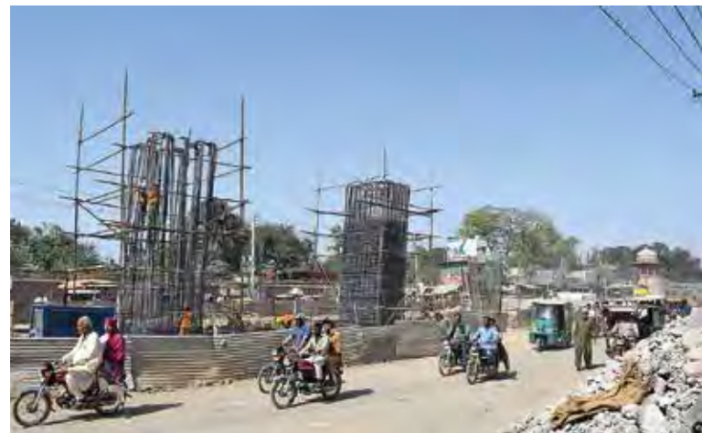
Construction of viaduct piers in front of Shalimar
