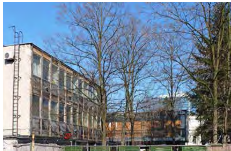
The smaller cube, much more modest and intended to house the museum's management (photo 2016)
