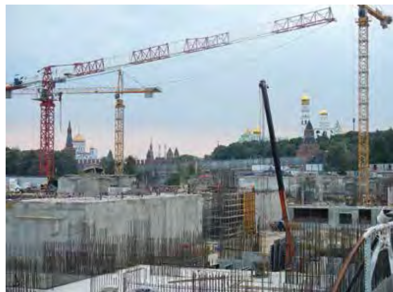
Zaryadye construction site
