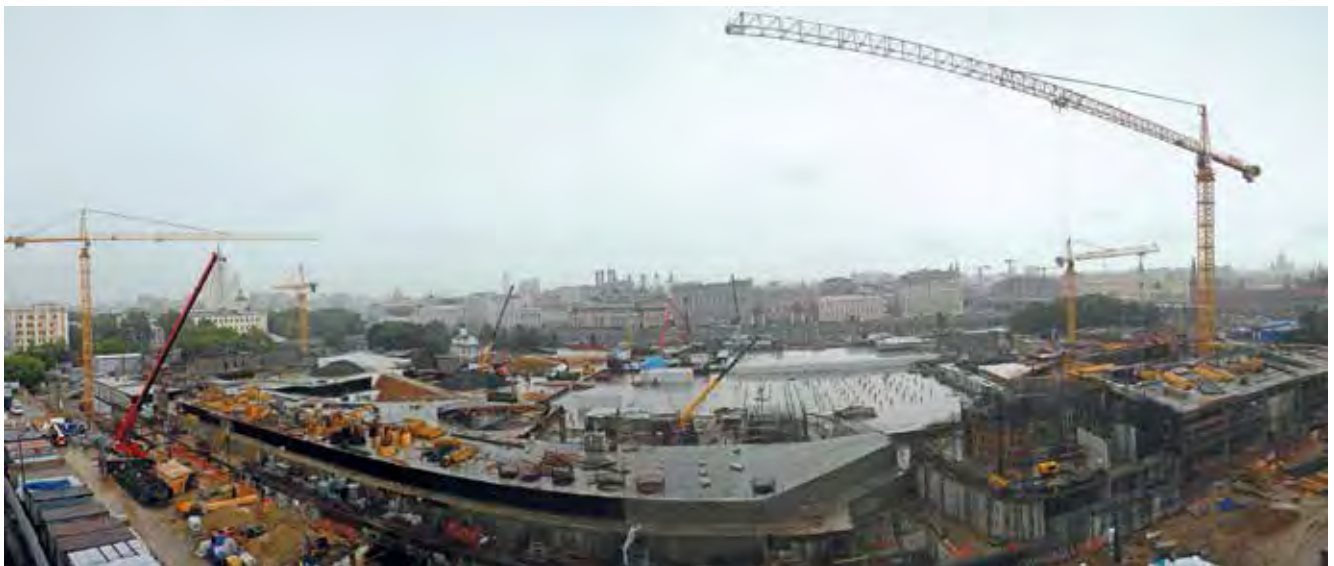
General view of the Zaryadye construction site
