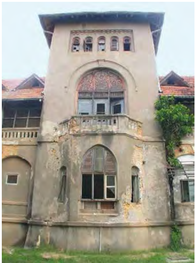
Oriel window at the rear side
