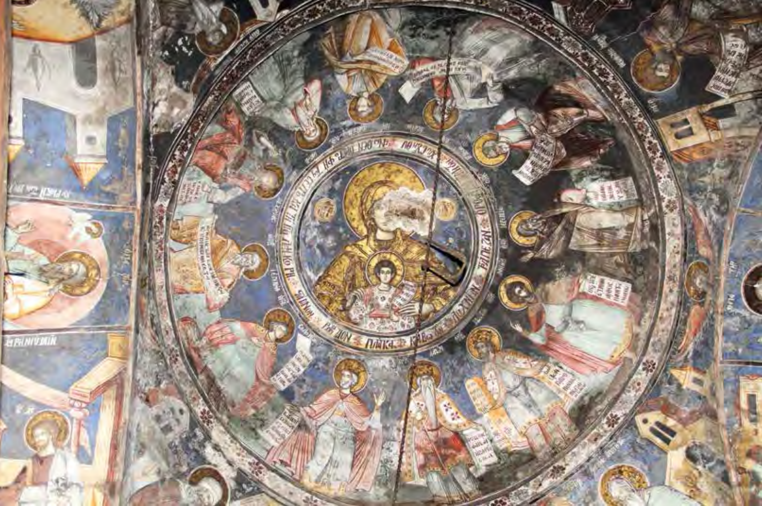
St. Athanasius Church, loss of the preparation and paint layers in the central cupola
