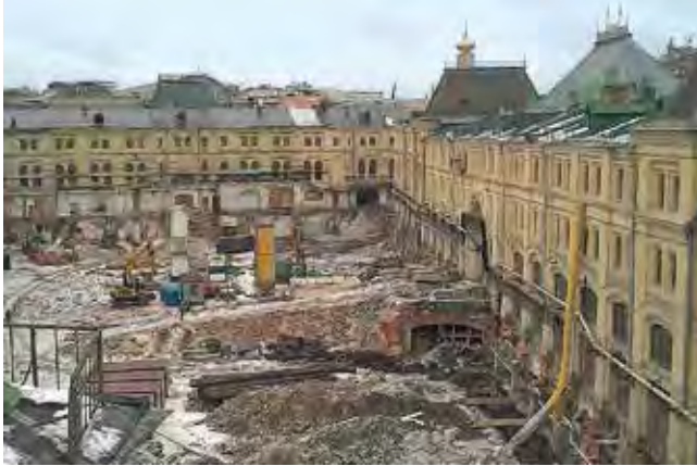
Demolition of the inner buildings of the middle rows
