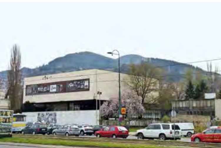
View of the Historical Museum's rear façade with garden (photo 2016)
