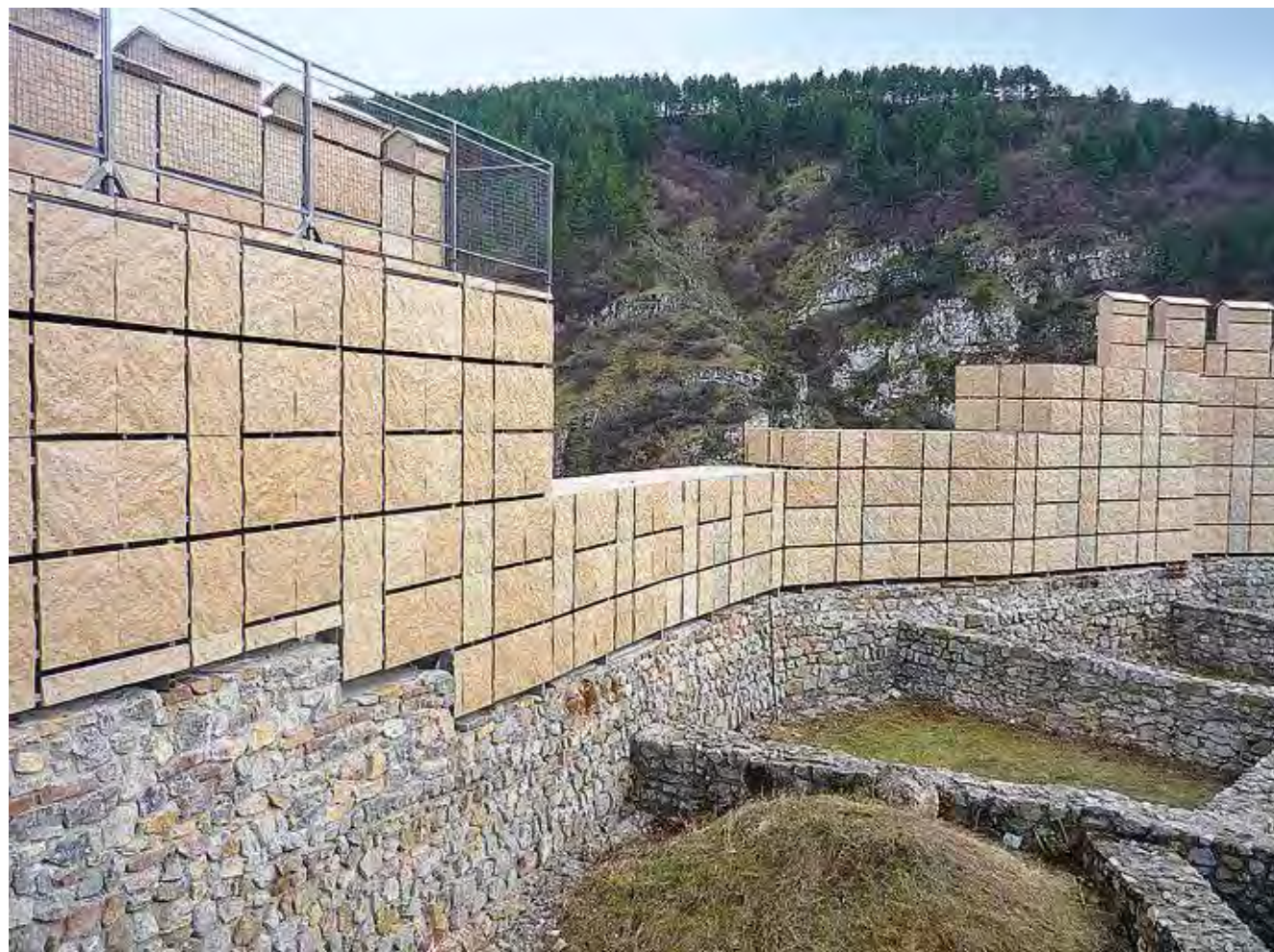
Ongoing reconstruction at Krakra fortress, Pernik
