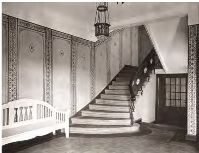
Historic view of the foyer, 1913 (photo Hamburgisches Architekturarchiv, Slg. Koppmann)
