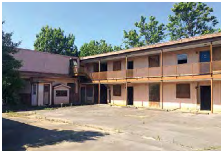
A.G. Gaston Motel in Birmingham, AL, (photo City of Birmingham Archives)
