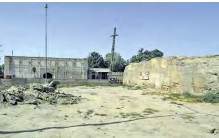
Shalimar Gardens and hydraulic tanks on GT Road
